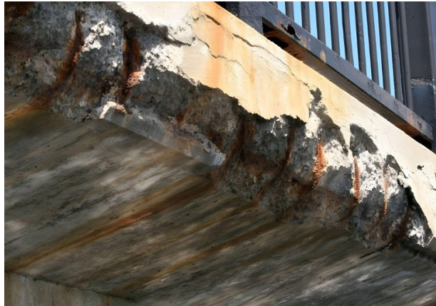
Ramsey County Bridge
